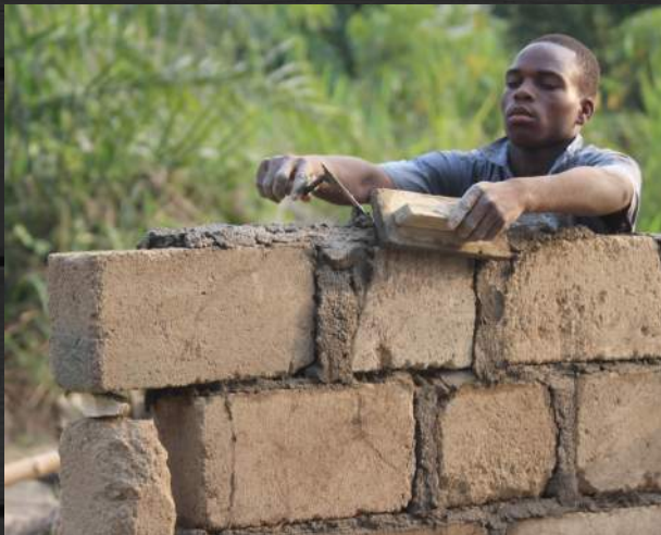
We always try to keep it local, so we made hand-mixed mortar using river water.
