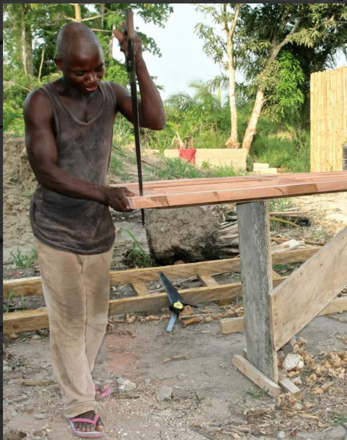
Building with sporadic electricity means no power tools. A hand sander and a hand saw were used to perfect the doors.
