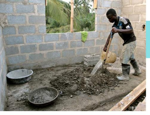
stone, sand, concrete, and river-water mixture used to fill the iron rods
